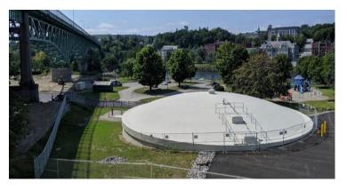
Typically, an underground tank made of precast sections linked together is utilized for CSO projects. However, the project team recognized that a tank normally used for drinking water storage could store combined sewer overflow at a very significant savings. The project was also able to provide additional site parking and standby power to the entire District campus and relocate a 1963 era pump station out of the flood zone.
