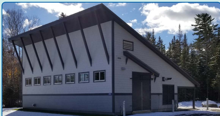
CVSD's main pump station was recently upgraded by TBuck Construction and Olver Associates
