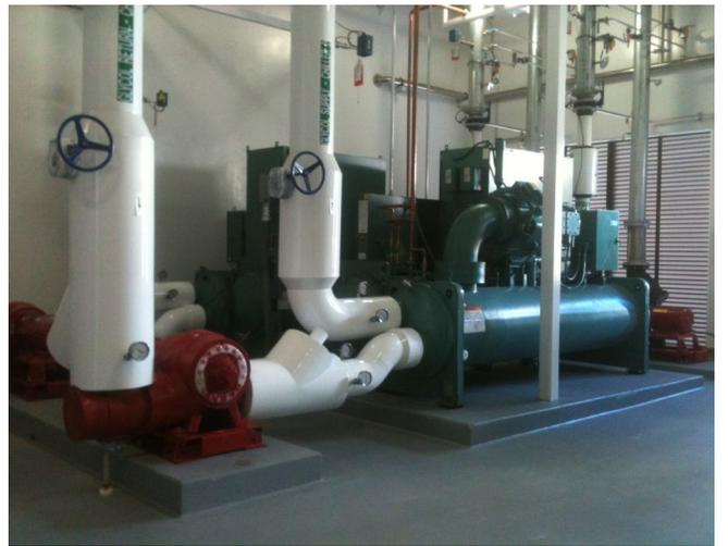
If possible, consider changing to a closed-loop system with a cooling tower, or otherwise, integrate the compressor cooling with another chilled water loop, like fermenting cooling. This chilled water loop is particularly effective when the brewery has several water cooled units. A small bleed will be needed for hygiene reasons.
