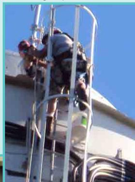
As February passes, we have removed the existing Healy-Ruff SCADA panels, reused their existing stainless steel cabinets and have installed the new non-proprietary PLC panels, narrow band frequency radios, and battery backup systems. We will be working with the radio vendor and consultant as we gear up for the programming of the radios and PLC's as well as the Master Controller Poll at the WPCF.
