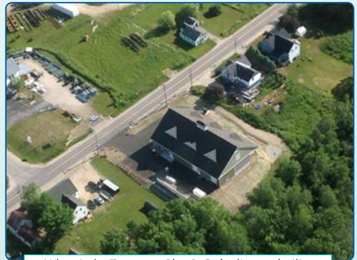
Where's the Treatment Plant? Oxford's new facility blends into the neighborhood.
