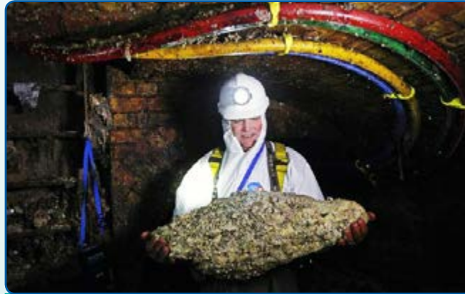
A sewer technician holds a "fatberg" as he works under London in December 2014. Photograph by Adrian Dennis, AFP, Getty Images
