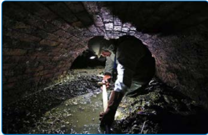
A technician shovels fat out of the London sewers in 2014. Photograph by Adrian Dennis, AFP, Getty Images
