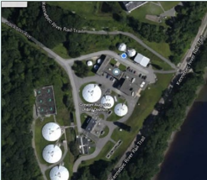
Aerial view GAUD WWTP
