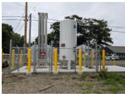
This supersaturated stream is bled into the pumped wastewater flow to help maintain DO in the wastewater through the force main. Official startup of the system was at the end of July. According to Tim, they have seen an extreme reduction and often elimination of H<sub>2</sub>S odors. Trials will continue over the summer.
