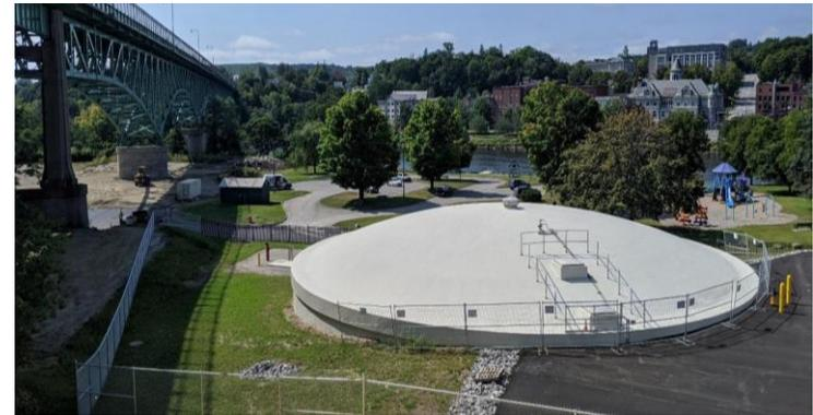
Typically, an underground tank made of precast sections linked together is utilized for CSO projects. However, the project team recognized that a tank normally used for drinking water storage could store combined sewer overflow at a very significant savings. The project was also able to provide additional site parking and standby power to the entire District campus and relocate a 1963 era pump station out of the flood zone.
